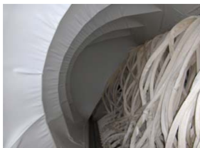
Drainage loops inside the tank
